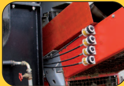
Quarrying – Greasomatics fitted remotely 5 metres away from the conveyor bearings
